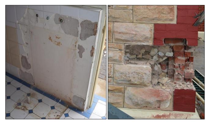
Figure 3. Damage with small flakes of plaster fallen from wall (already damaged by demolition works)
