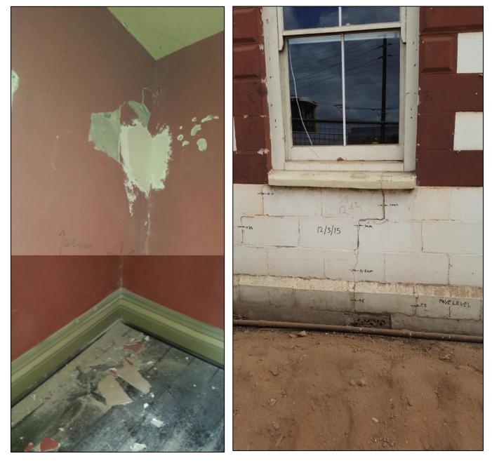
Figure 7. Cracked plaster (wall) and floor debris.
